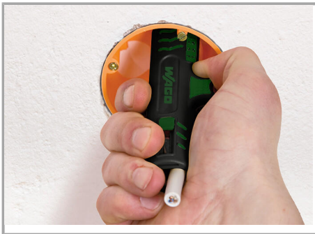
Stripping a cable sheath.
