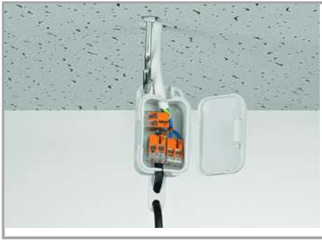
Pendant light connection in suspended ceilings
