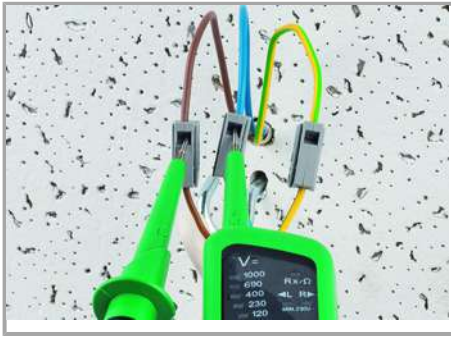
Testing via separate test ports.
