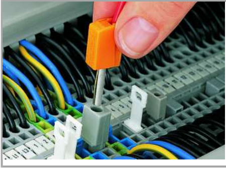
Testing with a test plug
