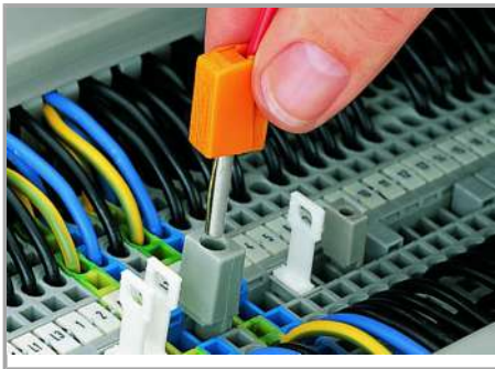
Testing with a test plug
