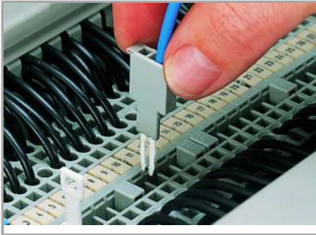
Testing with a test plug
