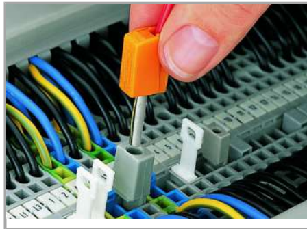
Testing with a test plug
