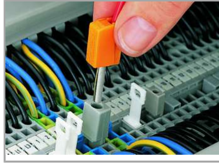
Testing with a test plug
