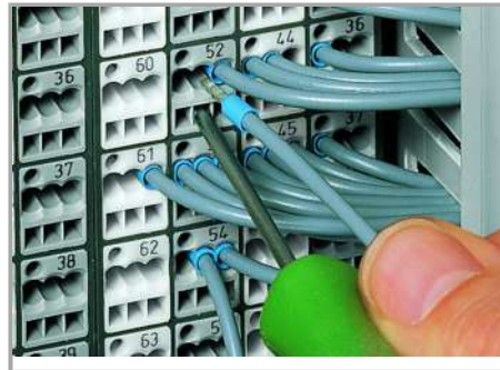
CAGE CLAMP® connection
