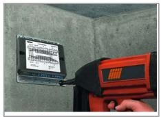
Securing the mounting plate with WINSTA<sup>®</sup> Distribution Box to the wall (e.g., via stud gun).
