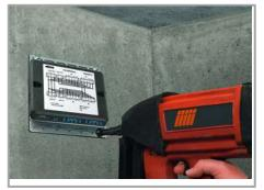
Securing the mounting plate with WINSTA<sup>®</sup> Distribution Box to the wall (e.g., via stud gun).
