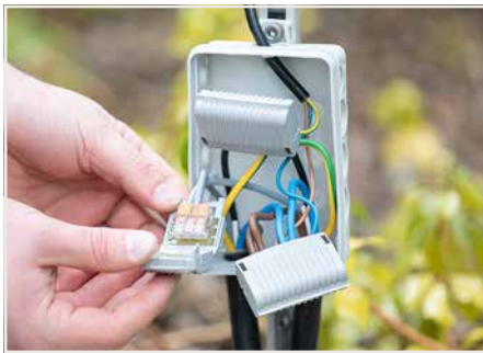
Connecting a bollard light
