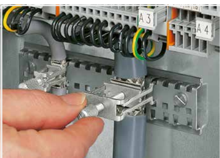
Tightening/removing a shield clamping saddle.
