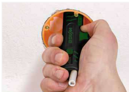
Stripping a cable sheath.
