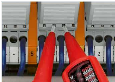
Function testing via touch-proof test slots.
