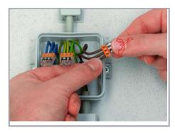
Removal: Hold conductor to be removed and twist alternately left and right while pulling the connector.
