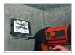
Securing the mounting plate with WINSTA  $^{\circ}$  Distribution Box to the wall (e.g., via stud gun).
