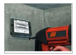
Securing the mounting plate with WINSTA  $^{\circ}$  Distribution Box to the wall (e.g., via stud gun).
