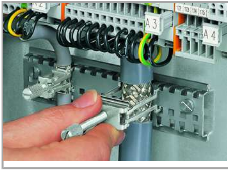
Fitting an additional clamping saddle.
