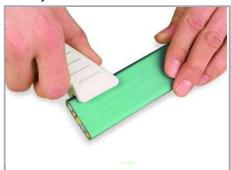
Cut both sides of the flat cable insulation using a stripping knife (observe 30 mm of cutting length).
