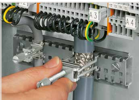
Securing an additional shield clamping saddle.
