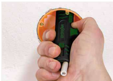
Stripping a cable sheath.
