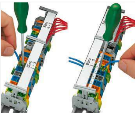
Laterally movable marking system
