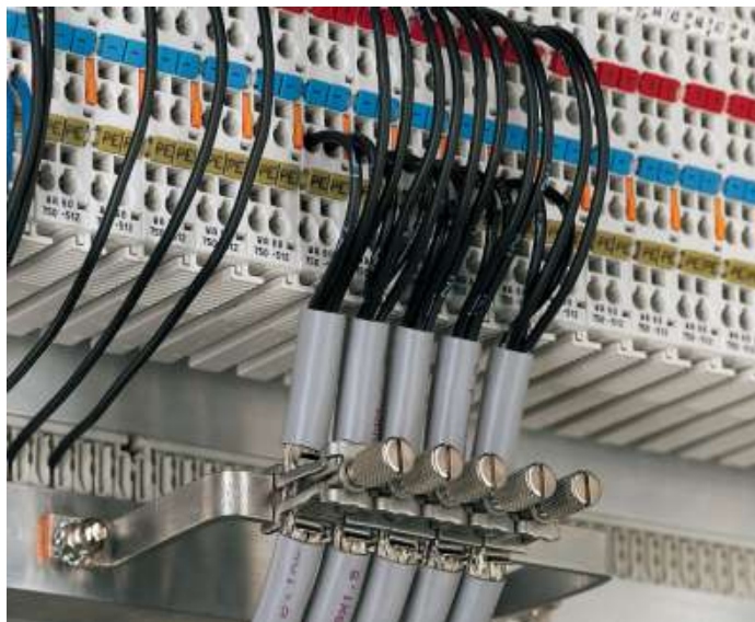
Figure 20: Application of the WAGO Shield (Screen) Connecting System
